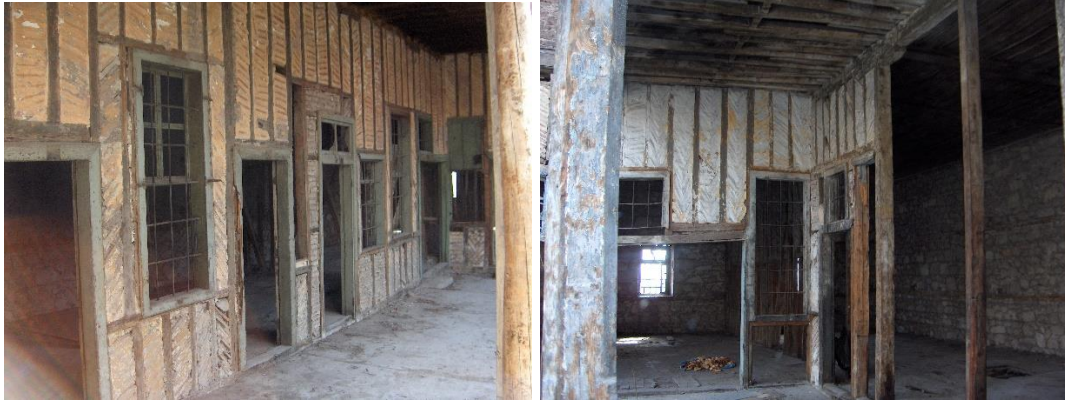
Figure 3. Wooden carcass system and the filling material (Archive of Ankara Regional Directorate of Foundations)
