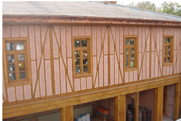
Figure 13. The room and partition walls of the upper floor have been renovated (Archive of Ankara Regional Directorate of Foundations)
