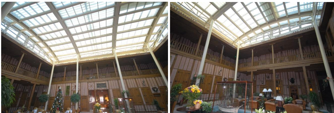
Figure 8. Courtyard top cover system (Archive of Ankara Regional Directorate of Foundations)
